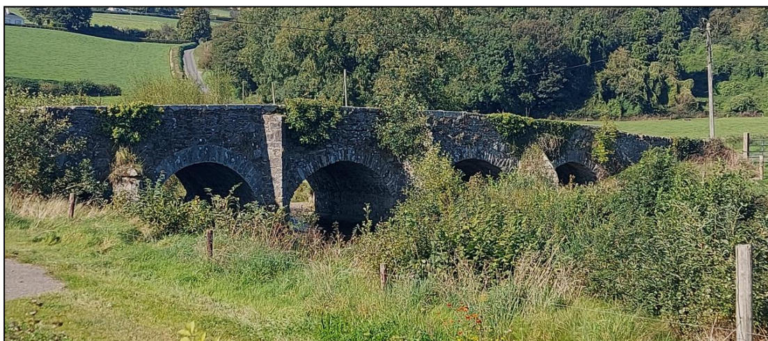
Plate 4.4.12 Stone Bridge Spanning the River Slaney
