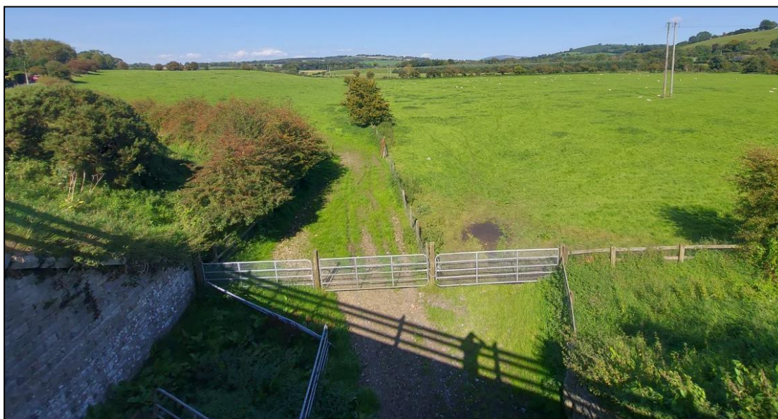
Plate 4.4.10 View of the alignment of the former Great Southern & Western Railway, from one of two overpass rail bridges
